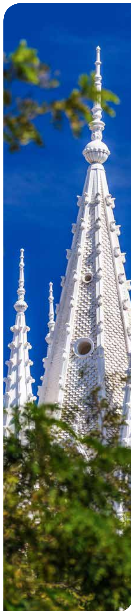
Tower of Santa Ana Cathedral, El Salvador
